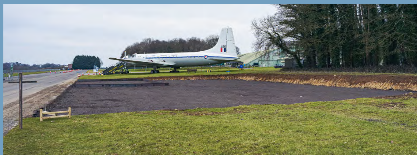
Concreted foundation laid at the future site for the BPAG's hangar, located beside the Bristol Britannia C.1 XM496 'Regulus'.
