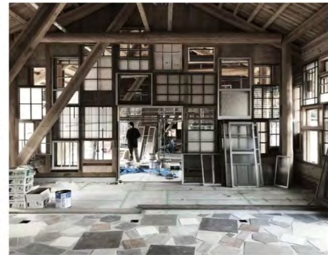
The wall comprises approximately 700 fixtures. On the floor of the lecture hall, we laid a medley of tiles that were headed for disposal, connecting their corners to harmonize the look.
