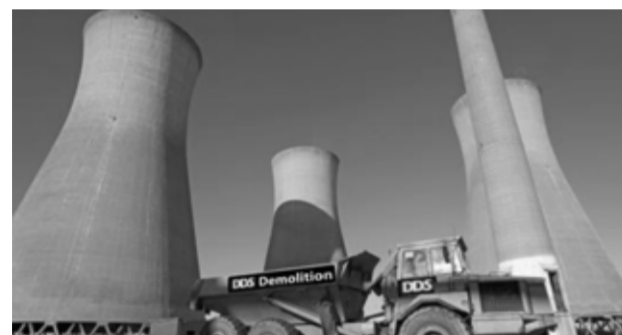
3. DDS demolition, Margate
