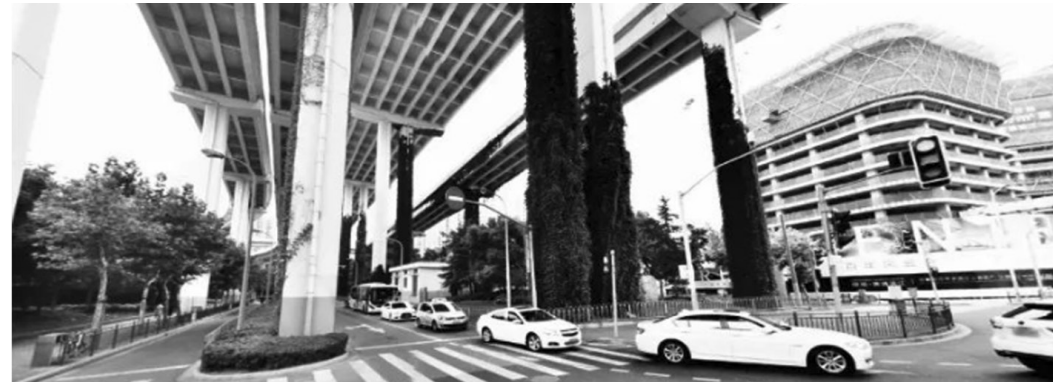
Figure 7.Space under the viaduct
