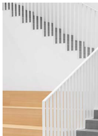
staircase close up
