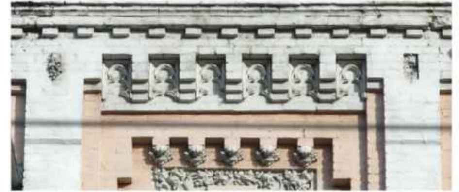
Brick facade with risalites, decorated with pilasters
