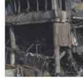
Reinforced concrete floor
