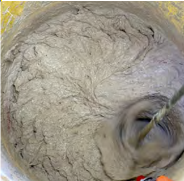
MIX PREPARATION cement . sand . aggregate
