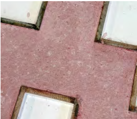
MIX POUR + SETTING carrera marble chips laid during setting
