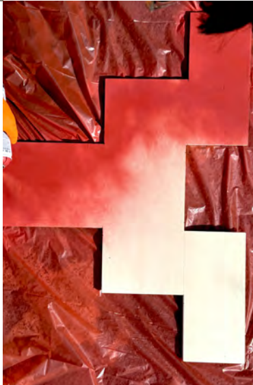
PAINT FINISH spray painted to mimic plaster finish
