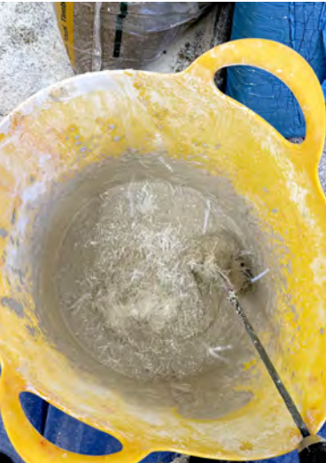
MIX PREPARATION cement . sand . aggregate
