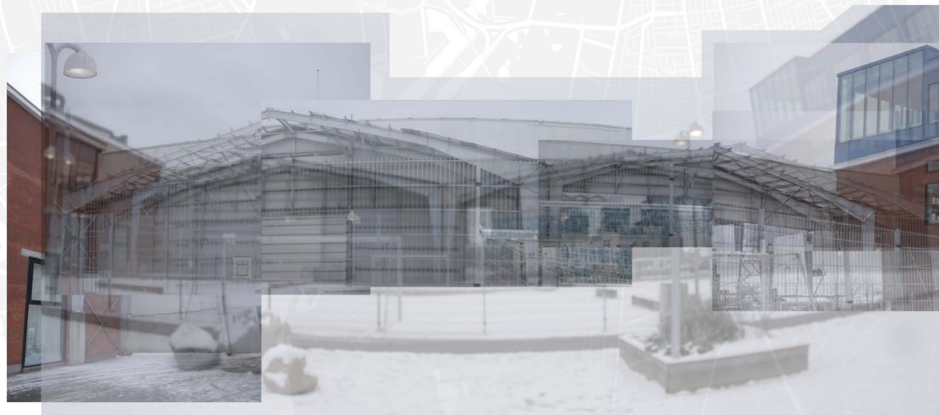
Site northern boundary and elevation [looking north]
