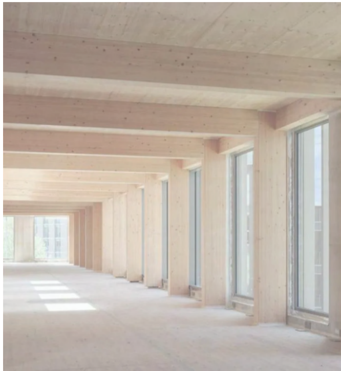
LVL & Glulam, CLT (Spruce) Structure, exposed internally
