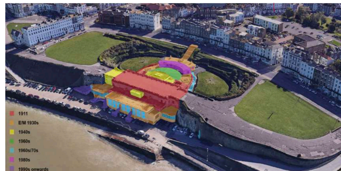
Fig.63: Winter gardens construction years
