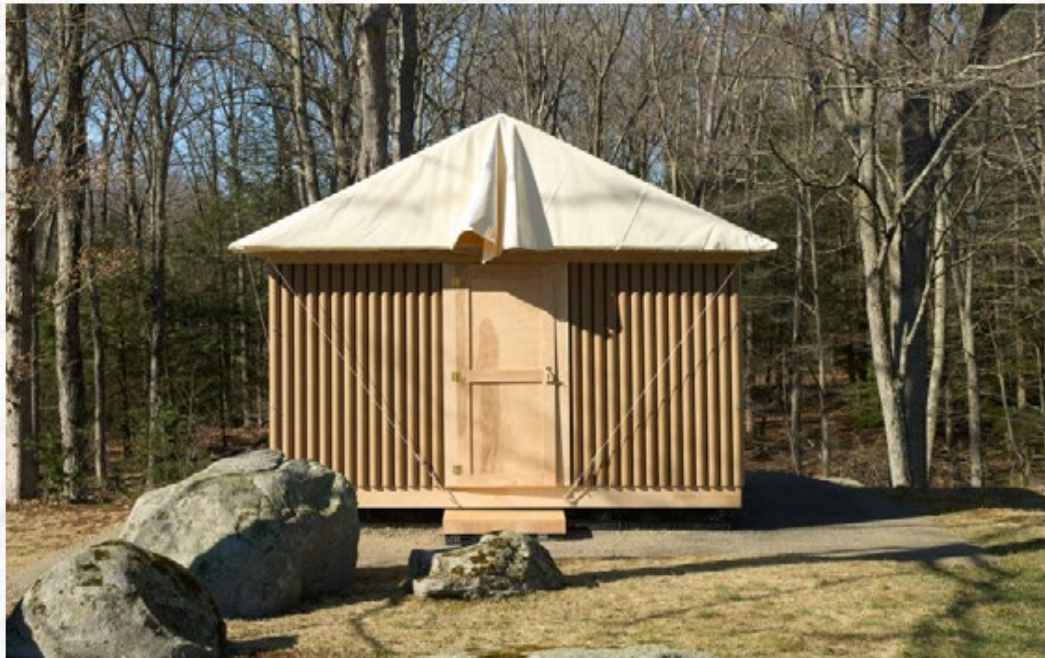
Fig. 94 The pavilion was made from paper tubes, wood and milk crates (2024)
