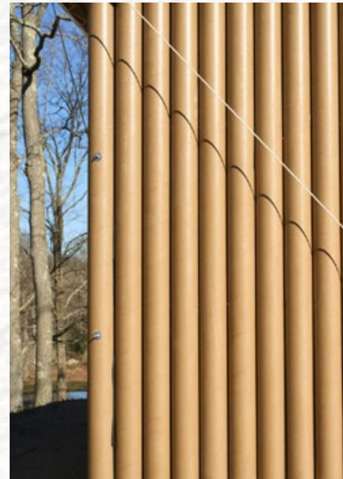
Fig. 95 Its structure contrasts the original house (2024)
