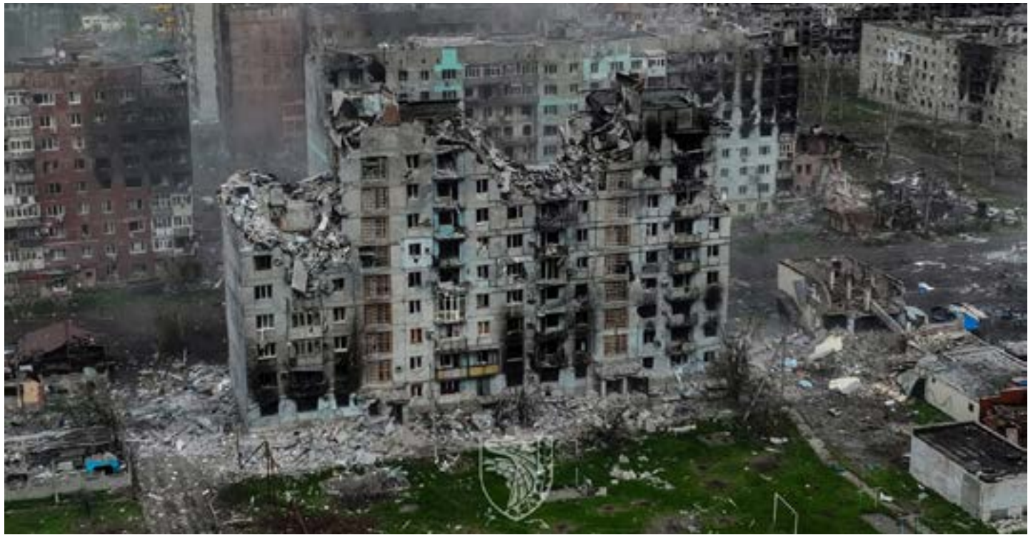
Destruction of Bakhmut city
