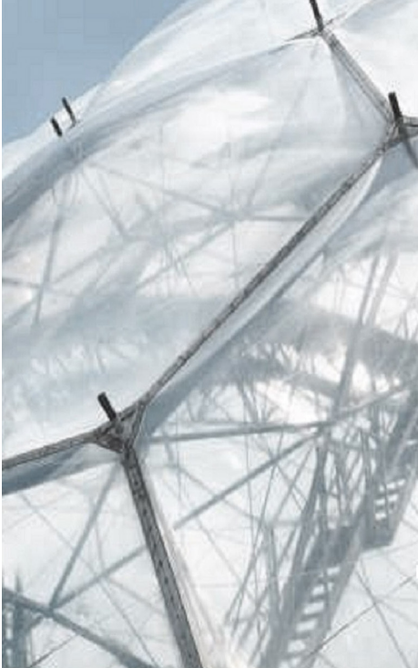
Fig.05 (left) ETFE Panels from the Eden Project
